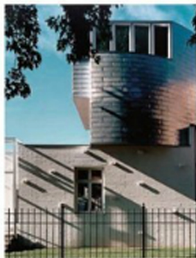
FRONT AND CENTERED From top: Architects Linda Searl and Joe Valerio's mixed-materials facade; street view of the residence.
